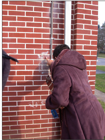
A property manager inspecting building exteriors for holes
