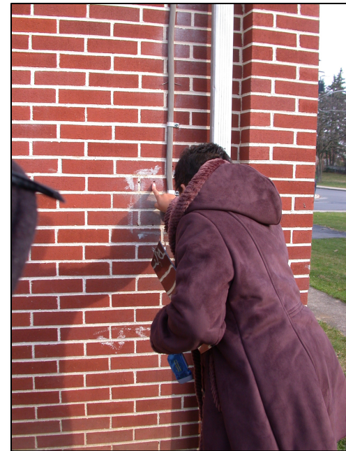
A property manager inspecting building exteriors for holes
